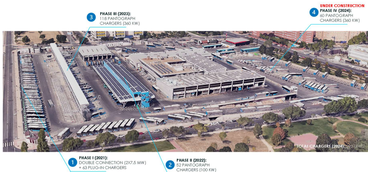
Figure 35. Aerial view of Carabanchel bus depot with the different electrification phases
