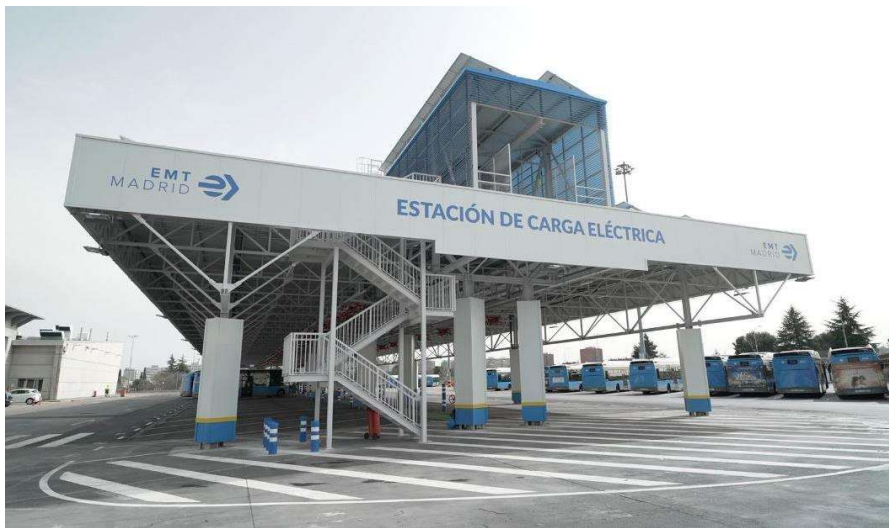
Figure 34. View of the first 52 inverted pantographs charging infrastructure for e-buses in Carabanchel bus depot (Phase II)
