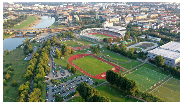
Figure 50. Ostra Area – Sports facilities (c) Landeshauptstadt Dresden / Jan Hübler
