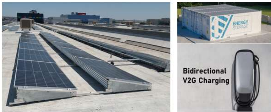
Figure 28. Example of rooftop PV panels, storage systems and V2G charger 2
